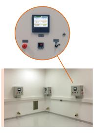
The whole system is supervised by Lumel-process program that allows remote process control and archiving of measurement data and creation of reports from the data.
